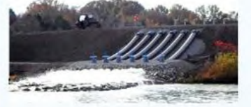
Pond A Spillway Improvements, Outer View Post-Construction, 2014
