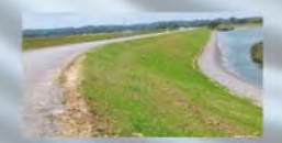
Pond A Divider Dike Improvements, 2014
